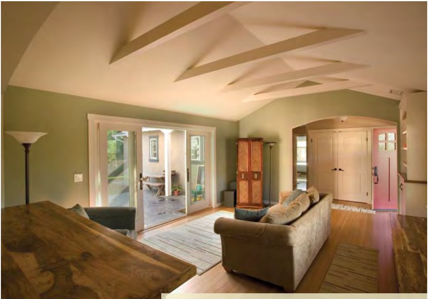
The new cathedral ceiling adds a feeling of spaciousness while a new French door adds warm sunlight to the remodeled living room.
